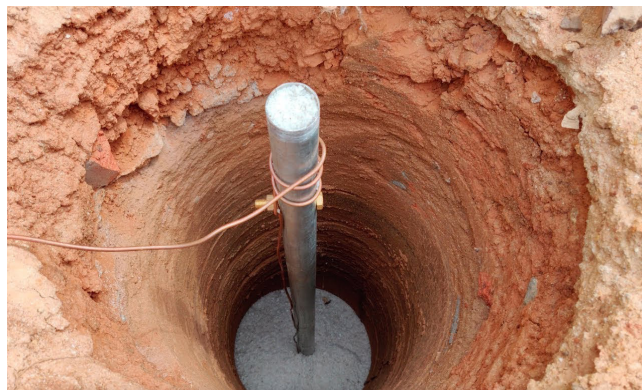
Fig. 4.2.2: Earthing device
