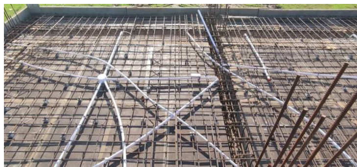
Fig. 4.1.13: Concealed Conduit in Slab
