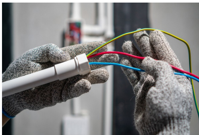
Fig. 4.1.19: Cable pulling
