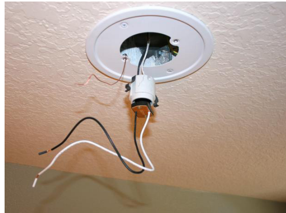
Fig. 4.1.17: Wiring and fitting fixture
